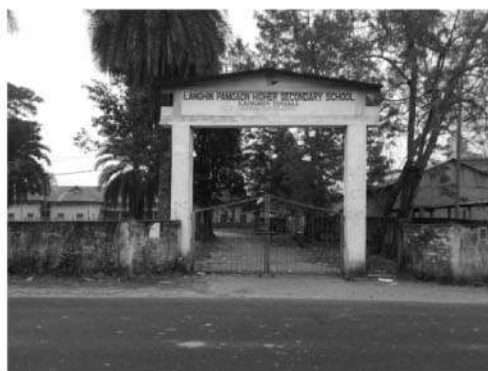
Figure 2.4 Langhin Pamgaon Higher Secondary School Hostel
