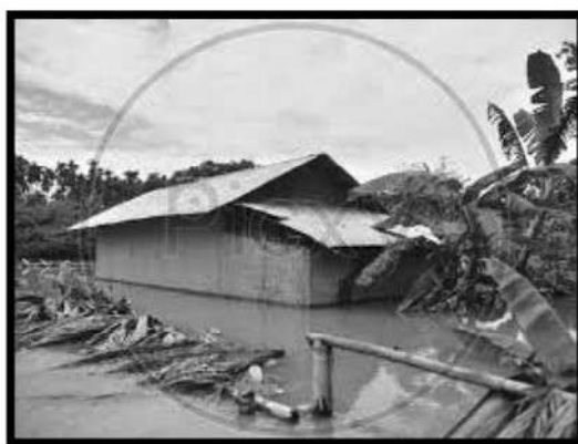
Flood Affected Hojai Village
